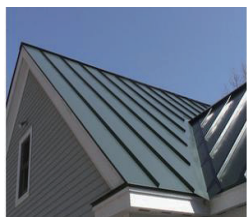
B. on the roof
